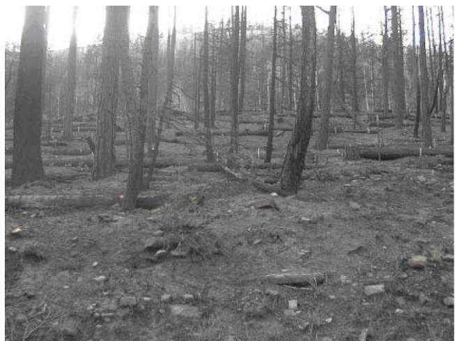
Log erosion barriers keyed into a burned slope at Lemon Dam. To work effectively, logs must be placed on contour with the topography and with good ground contact to inhibit undercutting by flowing water.
