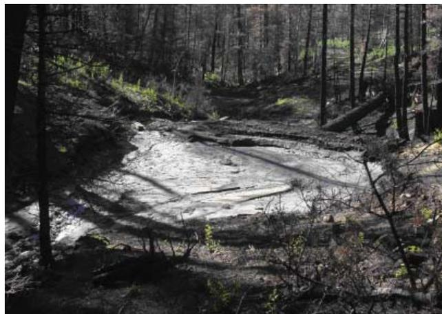
In order for check dams to function in collecting debris, they must be properly keyed into the banks of a channel. Weirs in the center of each dam allow excess water or debris to pass. When positioning check dams in the upper reaches—areas where debris flows begin in the burned landscape—the focus is on preventing materials from the channel bed from entraining.
