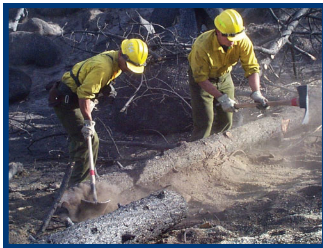
Figure 10.2 —Installing contour-felled logs for erosion control after a wildfire. (Photo by Peter Robichaud).
